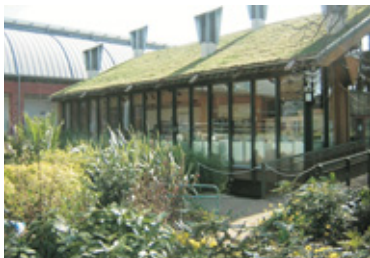
• Laban Dance centre London. This is a rubble biodiversity roof built to encourage Black Redstarts.
